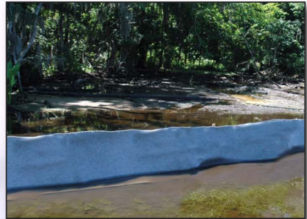
X-Tex used for Silt Fence
