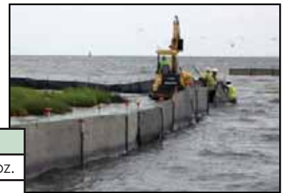
Ultra-X-TEX used for Spill Fence by Fore Construction
