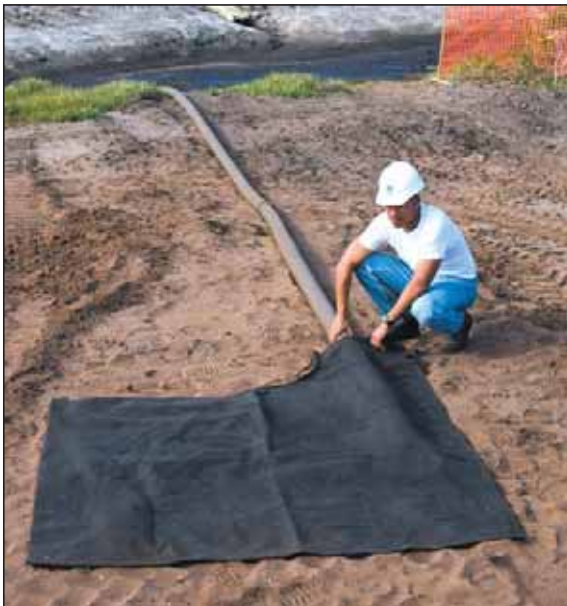
Ultra-Dewatering Bag — Contain Sediment and Oil During Dewatering Operations
